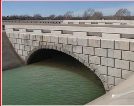
Loop 335 @ Amarillo Creek
