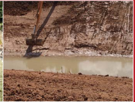
Eagle Landing - Channel Rectification
