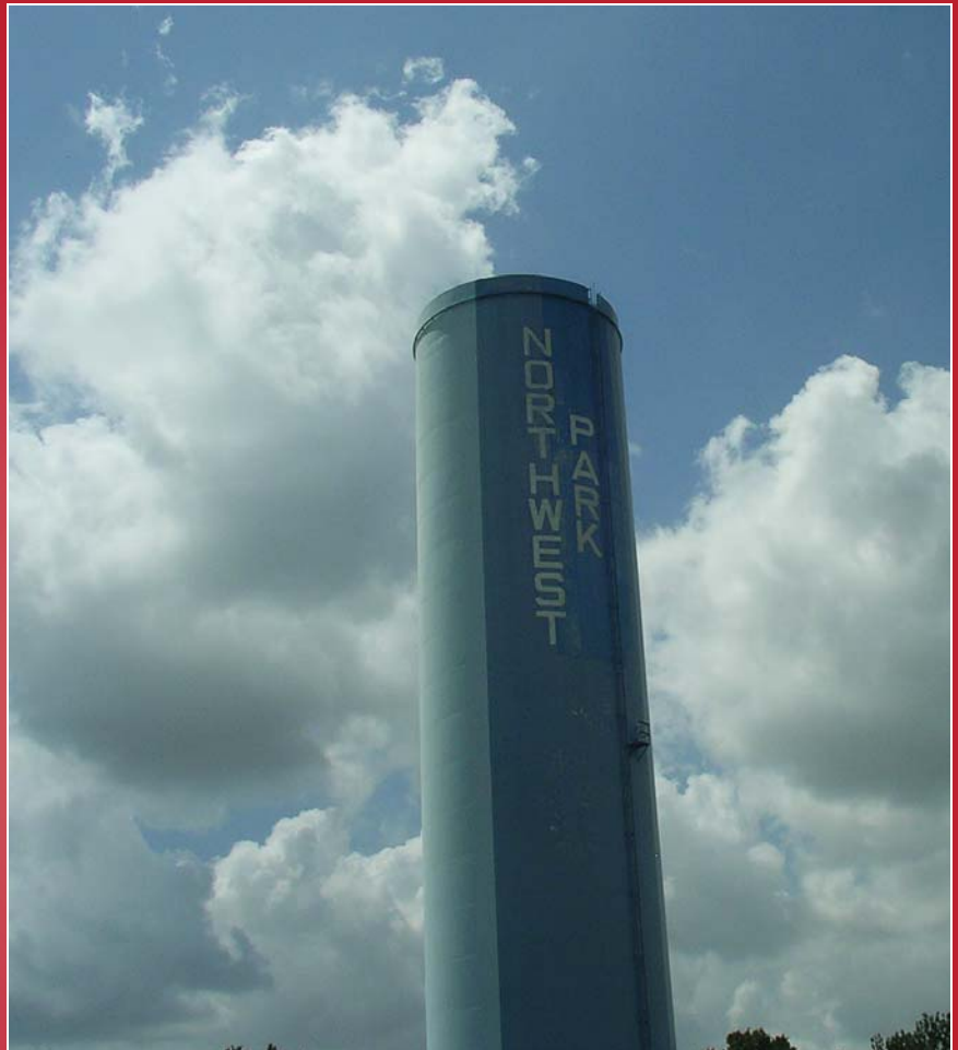
Northwest Park - Standpipe
