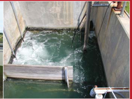
Williamsburg Regional - WWTP
