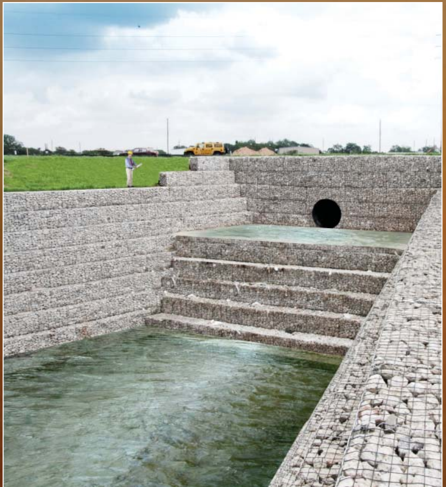
Gabion Outfall Structure at Rio Vista - Construction Monitoring
