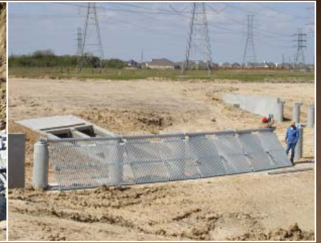
SWQ Structure Construction Monitoring
