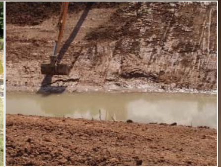
Eagle Landing - Channel Rectification
