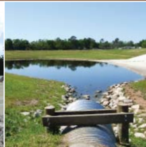
Brickhouse Gully Detention
