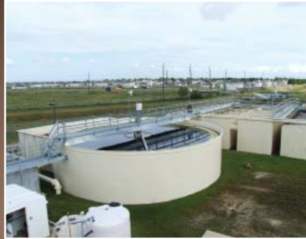
HC MUD No. 127 - WWTP
