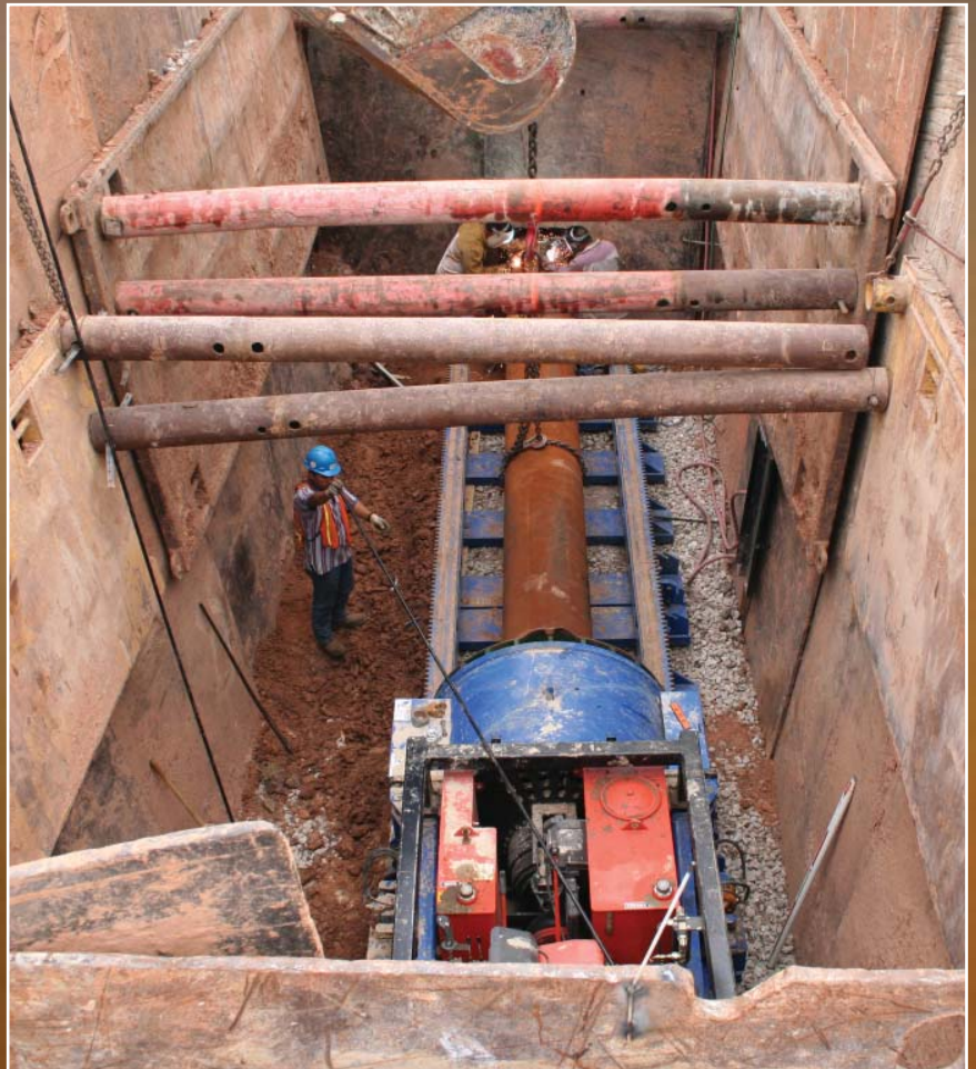
Rio Vista - FM 359 Trunk Utilities
