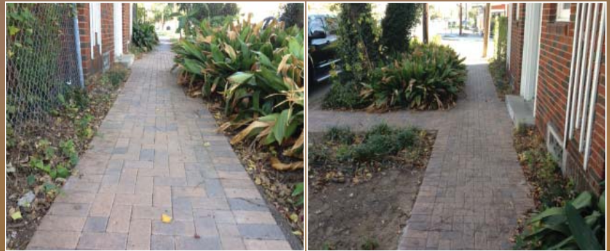
TIRZ 13 Sidewalk Rehab
