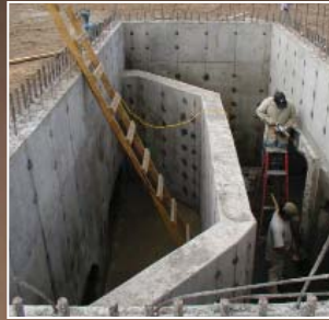
Junction Box - Towne Lake
