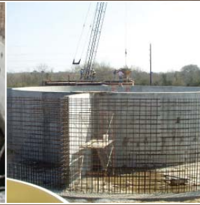
WWTP - HC MUD No. 127
