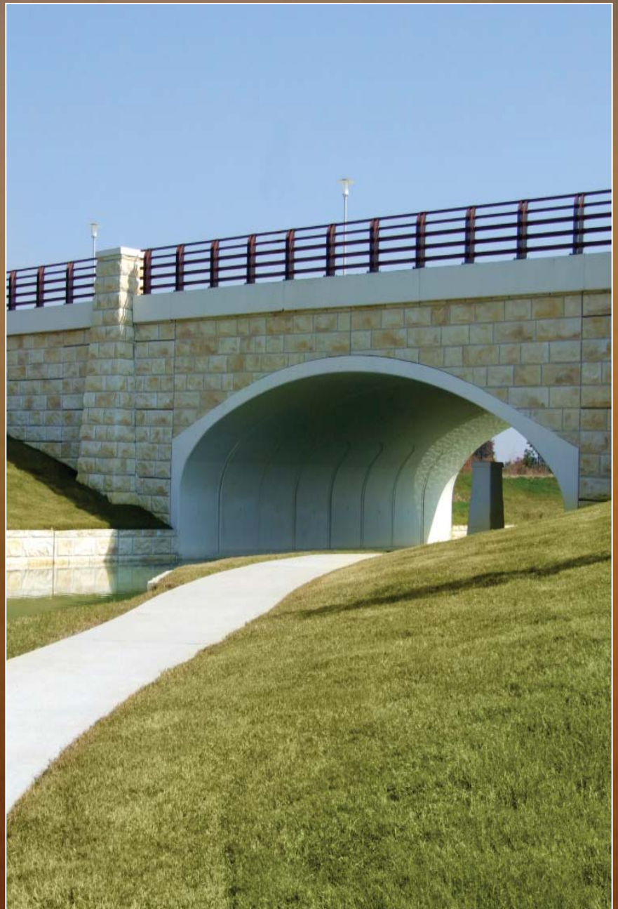
Concrete Arch Bridge - Hamilton Hills Road - Towne Lake
